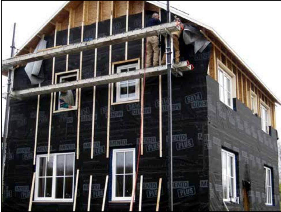
*House 7 with "1 Beam" construction permitting 12" of total outside insulation*
